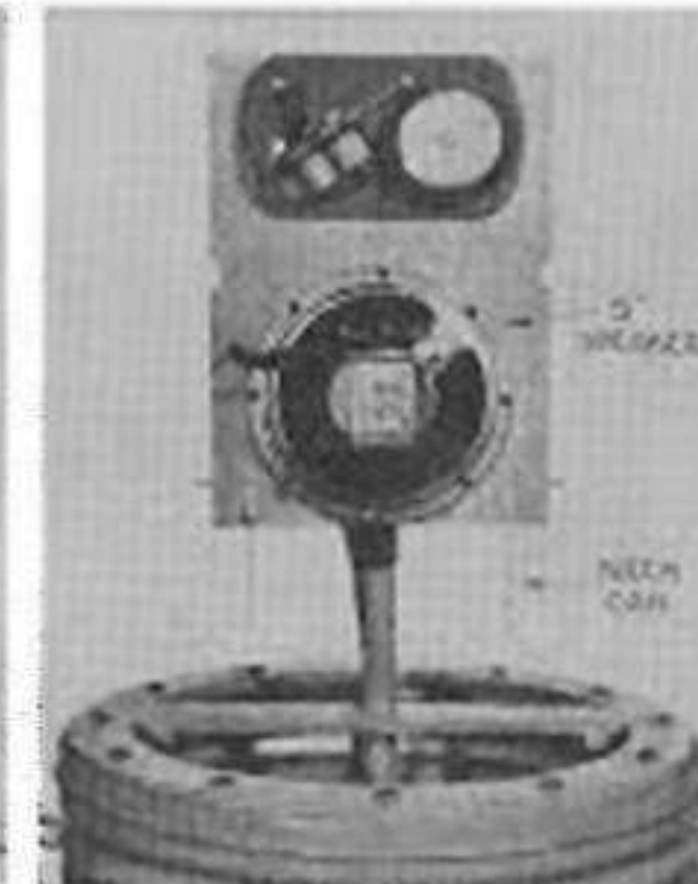
Back of headboard with bell and speaker. Notches clear ear screws.
